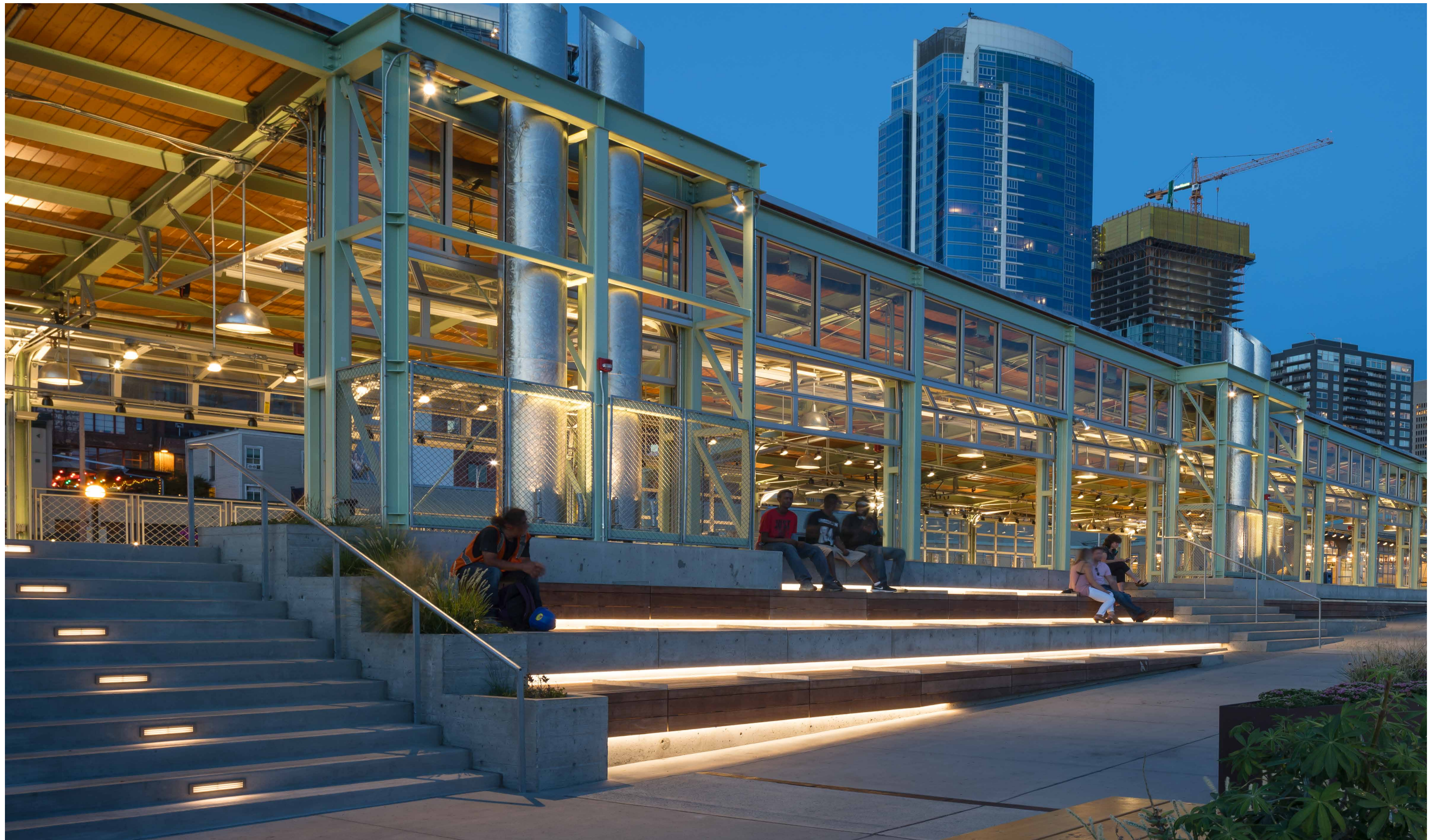
A layered approach to lighting creates safe and intuitive circulation at night. Site lighting is carefully integrated into vertical features below eye level so as not to distract from nighttime views of the waterfront.
