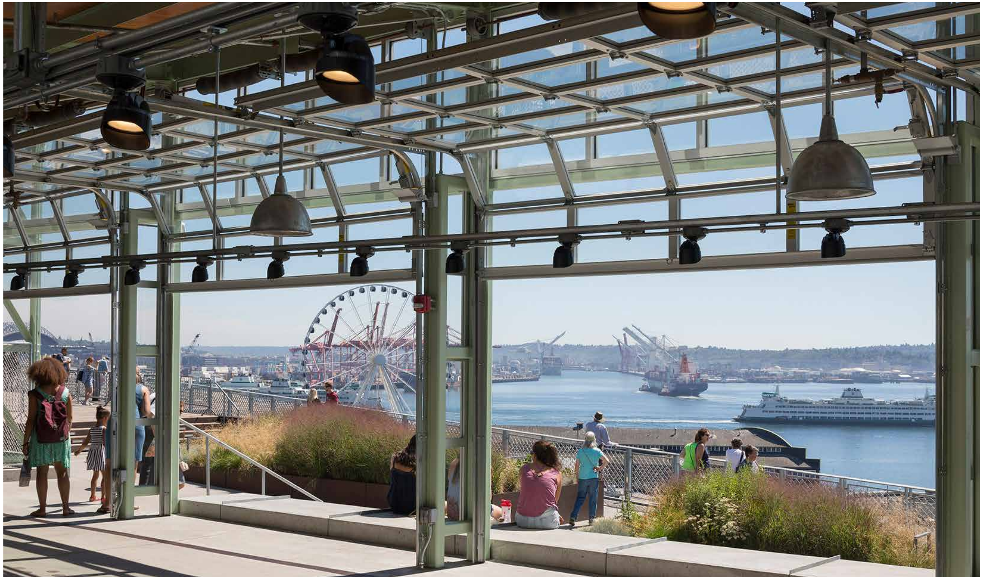
Market Stalls: A large pavilion anchors the Market Plaza and provides flexible, covered space expanding the Market's vendor capacity and creating a new venue for events. Incoming revenue supports the many social services provided by the Market.
