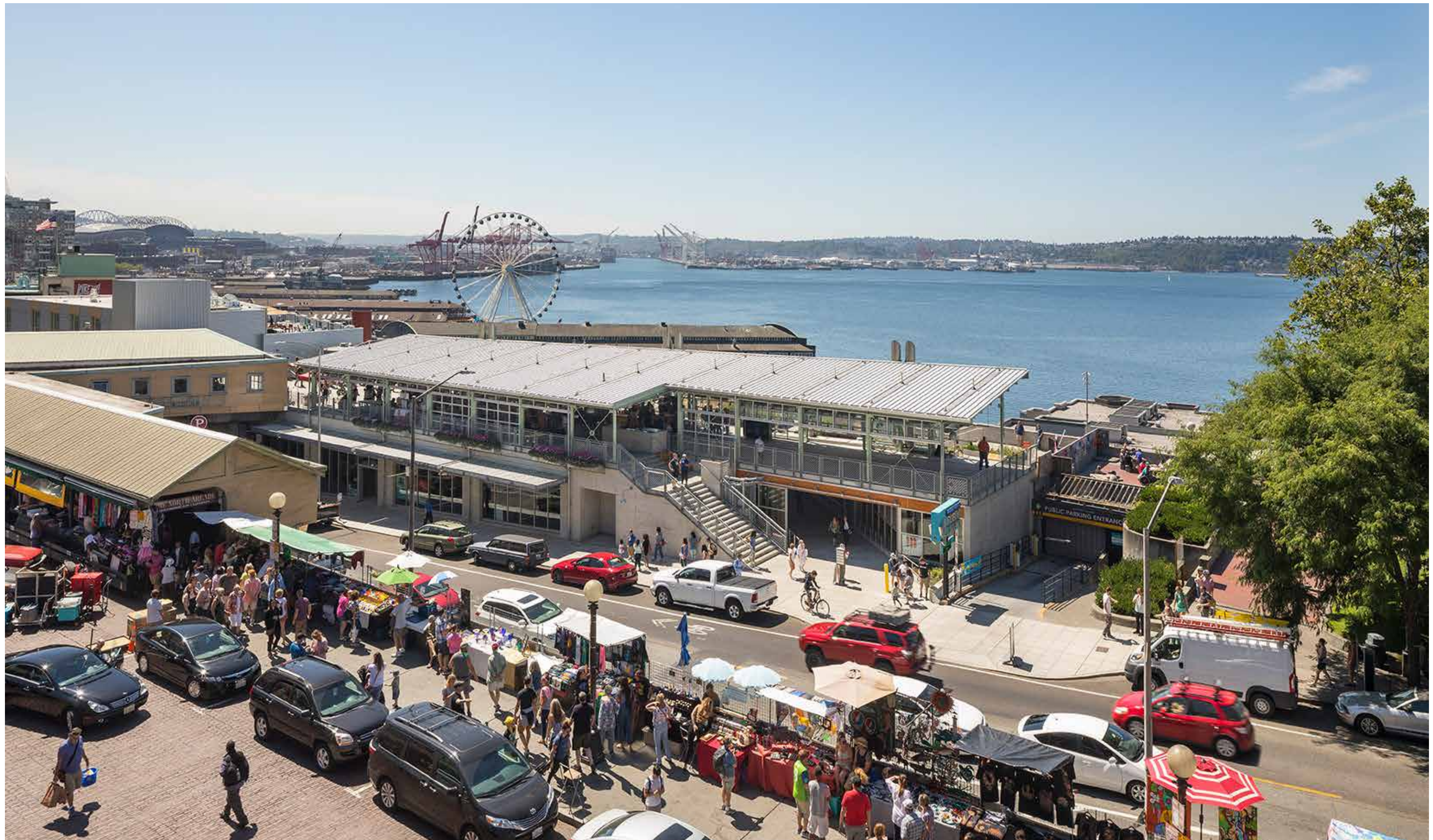
The Market's Historical Commission required viewsheds from Pike Place Market be maintained. Once the Hwy 99 viaduct is demolished, an entry portal through the building will provide ADA accessibility to the waterfront via the Overlook Walk (OLW).
